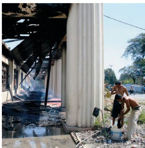
Destruction in the aftermath of the riots
