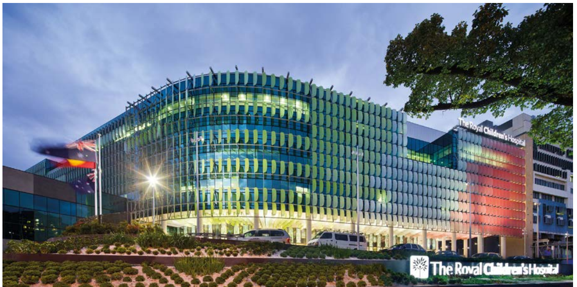
The Royal Children's Hospital, Melbourne. Photo by John Gollings
